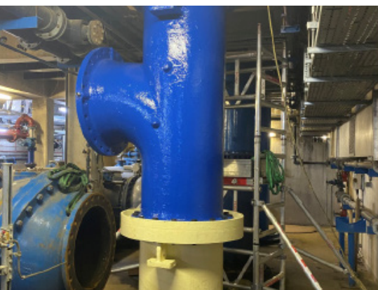
Refurbished and repainted pipework
